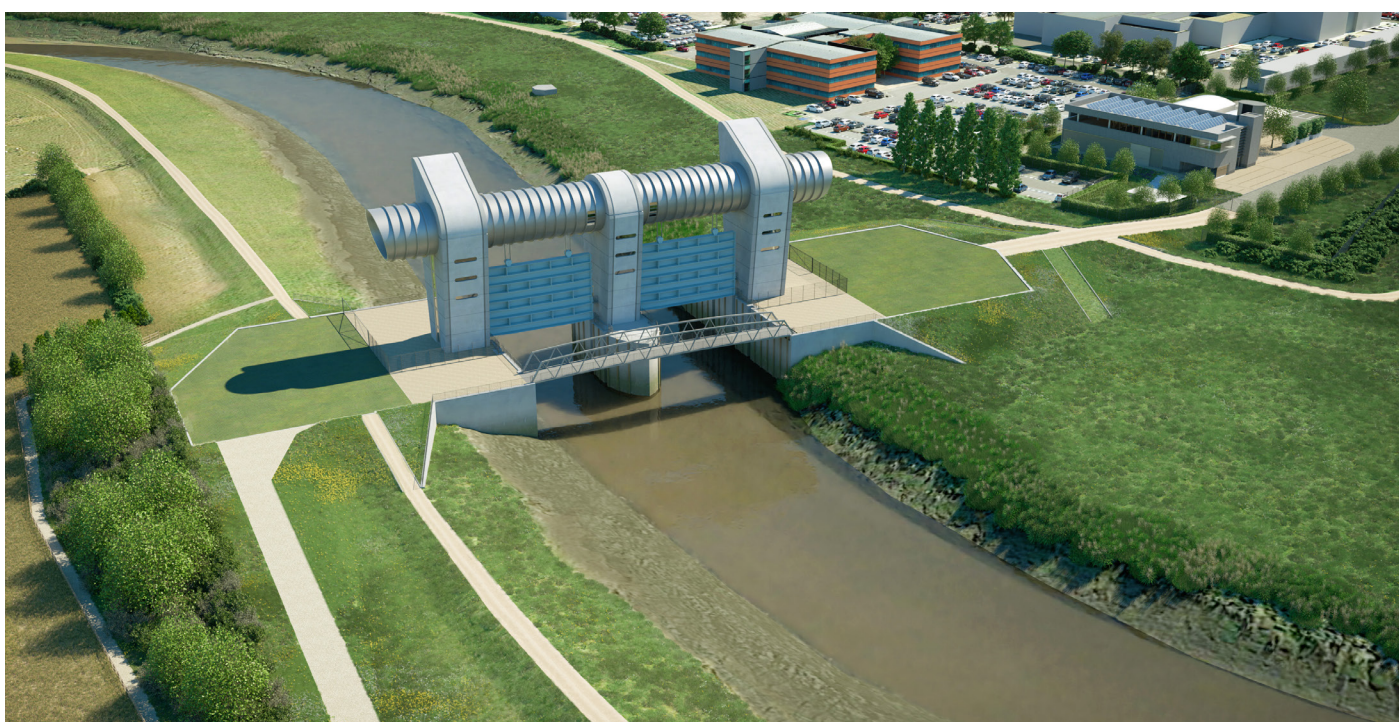
Bridgwater Tidal Barrier
